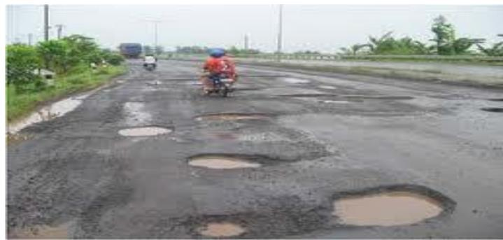
Gambar 3.3 Lubang (*potholes*)
