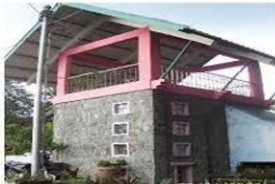
Lampiran 8. Power House
