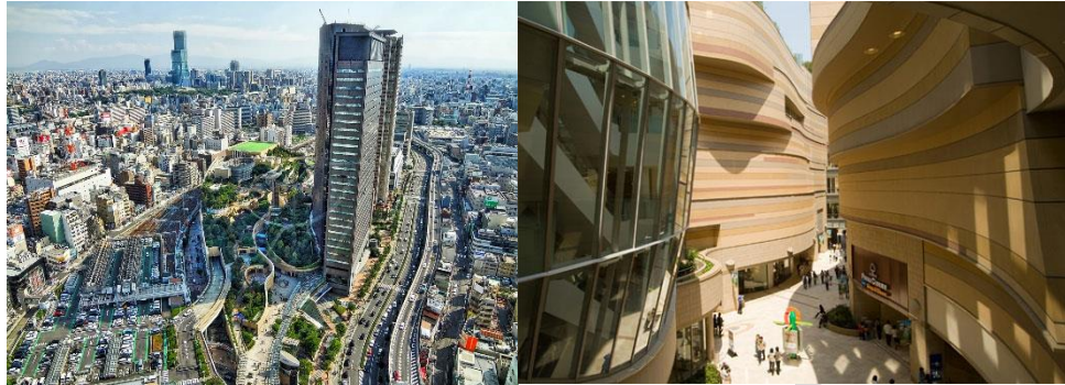
Gambar 2.13. Namba Parks Mall ( https://inhabitat.com/japans-namba-parks-has-an-8-level-roof-garden-with-waterfalls/ , diakses pada April 2018)
