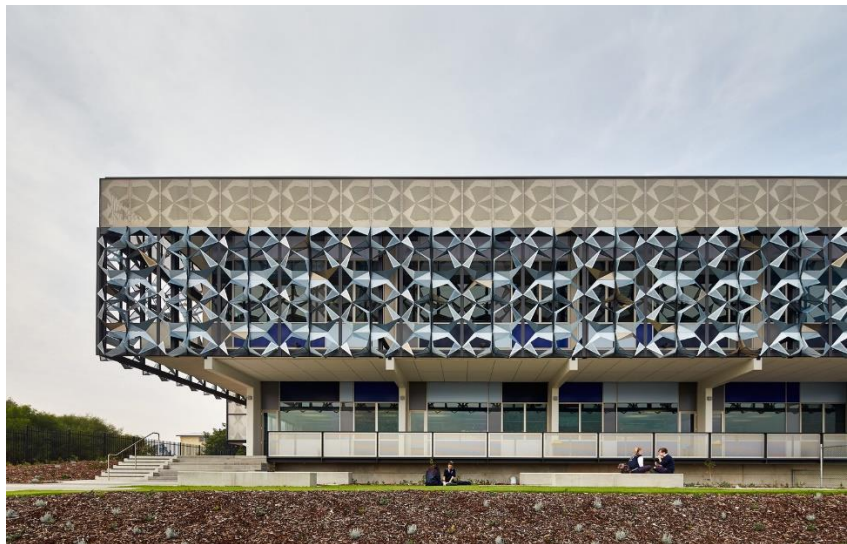
Gambar 2. 30 Fasad John Curtin College Sumber: Bennets, 2015.
