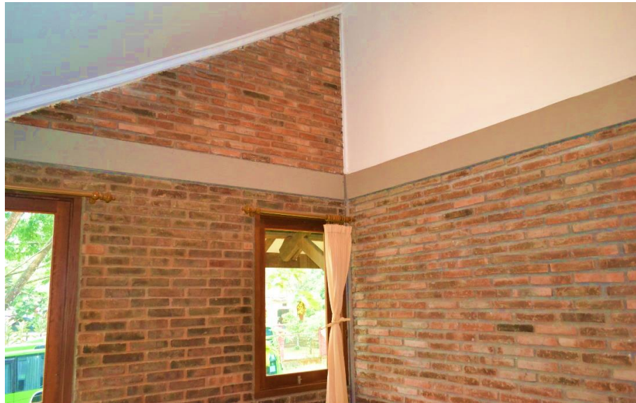
Gambar 3.12: Dinding Bata Expose
