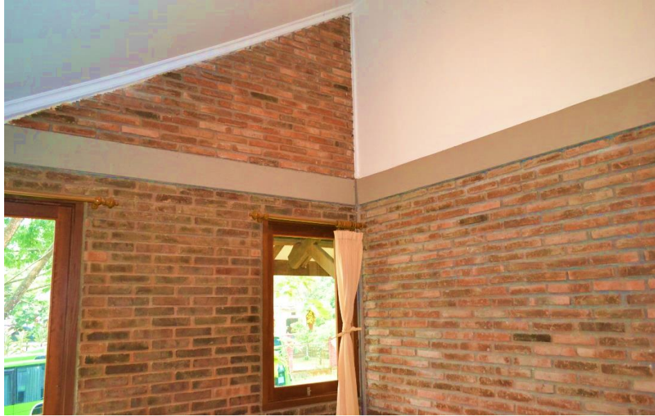
Gambar 2.7: Dinding Bata Expose
