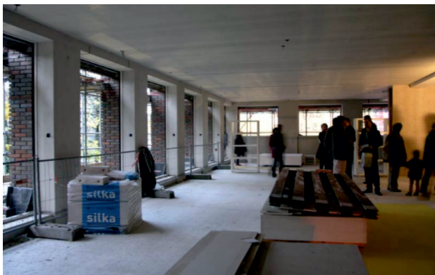
Gambar 2.23 Interior of Solid Oud West under construction
