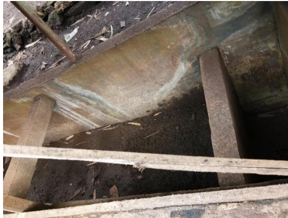
Gambar 4.4 Sludge Drying Bed Desa Pucanganom
