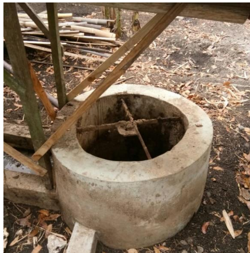
Gambar 4.1 Mixing Unit biogas Desa Pucanganom
