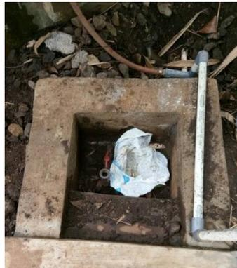
Gambar 3.5 Terminal pipa biogas
