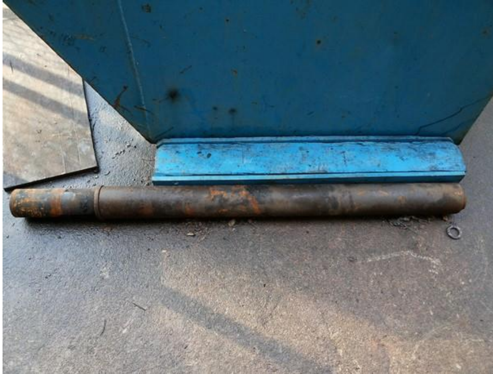
Lampiran 3. Head shaft patah (Sumber : PT. Kaltim Prima Coal)
