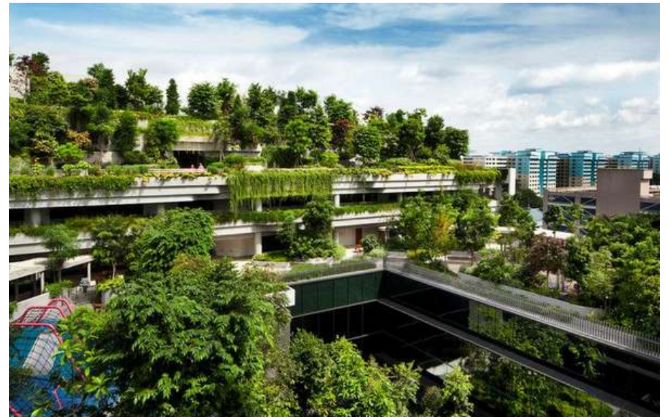
Gambar 2.28 Green Roof Kampung Admiralty Sumber : archdaily, 2017
