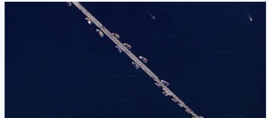
Figure 1.46 Boat parking in trestle bridge edge
