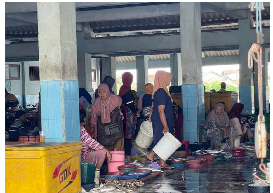
Figure 3.13 Existing Auction Building Condition
