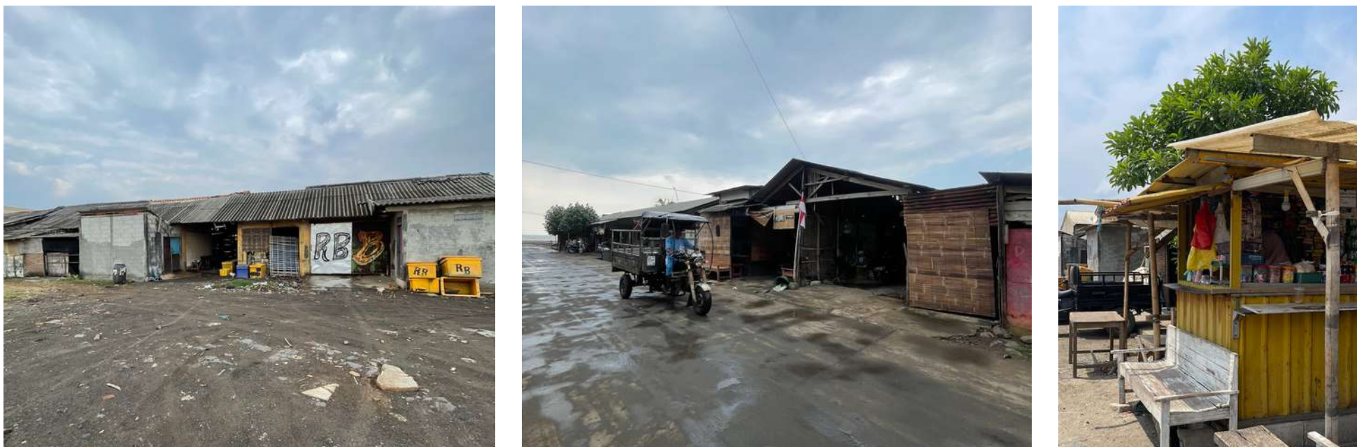
Figure 3.16 Existing UMKM Building Condition
