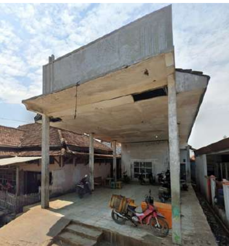
Figure 1.6 TPI Kedung Malang Source: Google maps perspective, 2025
