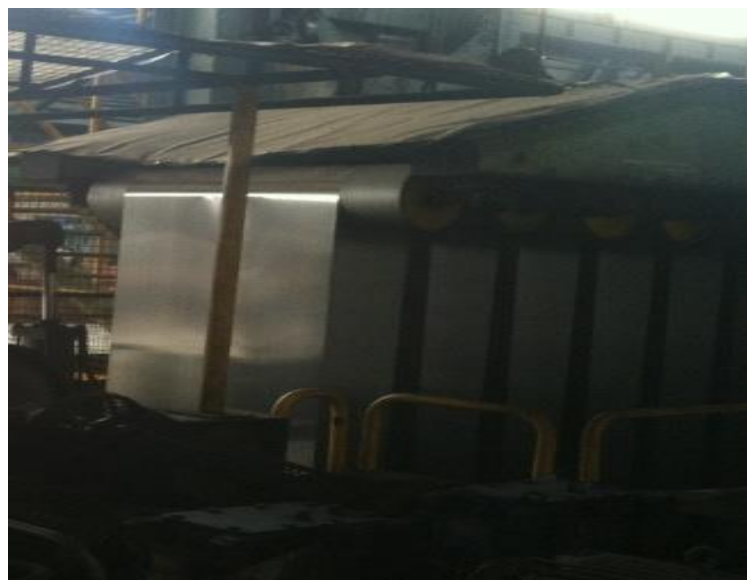
Gambar 4.6 Entry Loop Tower
