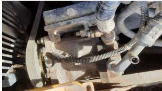
Gambar 4. 4 Klaim Compressor Broken
