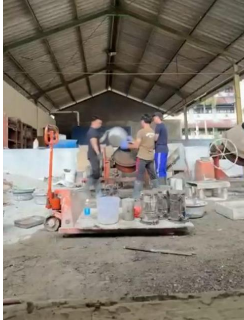
Gambar 7.1 Proses Mixing Beton
