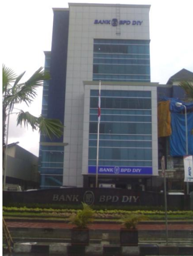
Gambar 5.1 Gedung Bank BPD DIY
