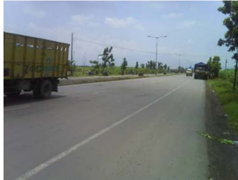
Gambar 4.50. Kondisi Lalu Lintas Jalan By Pass Kudus
