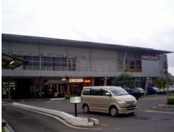
Gambar 3.5. Parkir Rest Area Km 19
