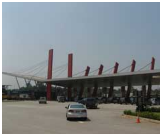
Gb 3.2. SPBU Rest Area Km 19
