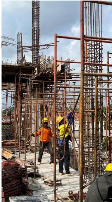
Gambar L-2.1 Proses Pemasangan Scaffolding
