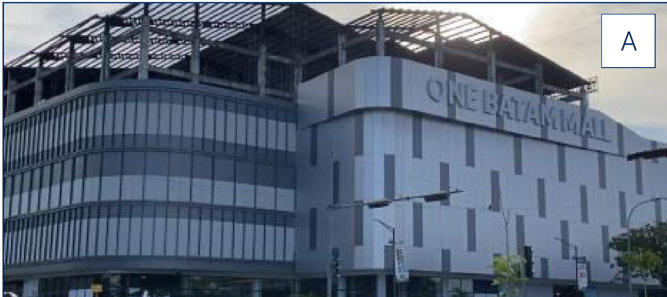
One Batam Mall 50m away from site Source: Author, 2025
