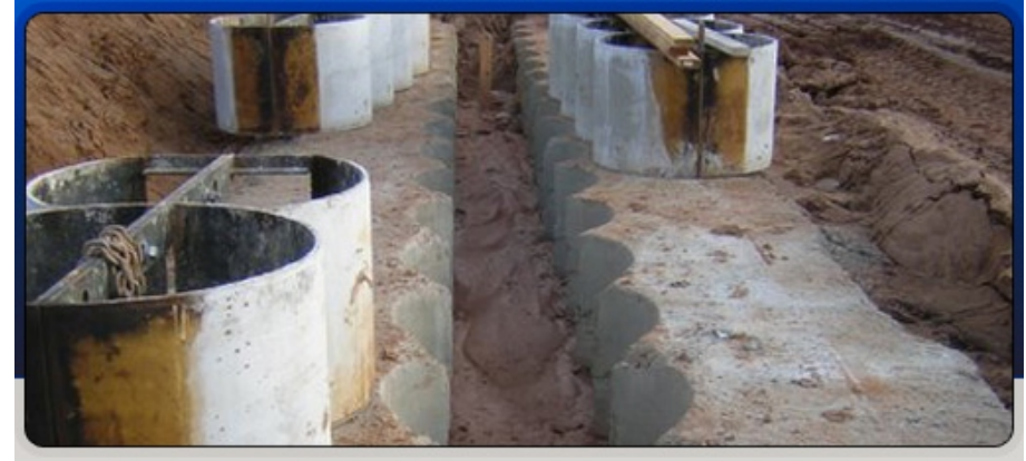
Gambar 24. Dewatering Cut off Sumber: http://tukangbata.blogspot.com/
