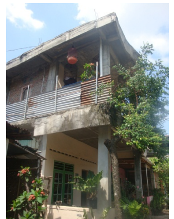
E Typical incremental growth of the house in high-density housing area : going vertical with the addition of new structure
