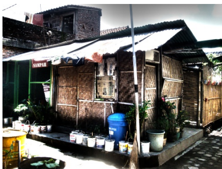
Fig 3.9 trash warehouse and central workshop Photo credit: author. Taken Sept, 2011
