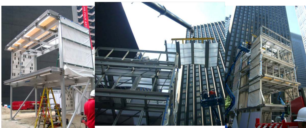
Fig 4.12 Set of Images : Cellophane House On Site Completion
