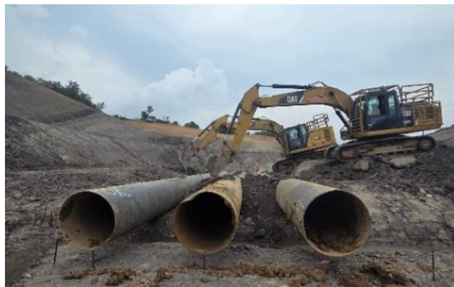
Gambar L-5.6 Penimbunan Pipa
