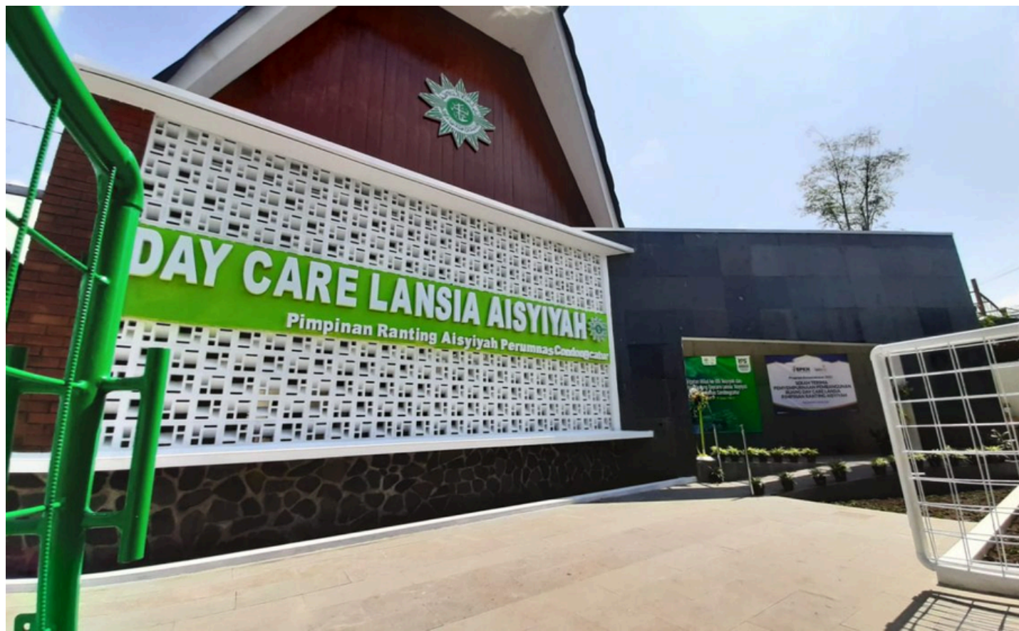
Gambar 2.4 Gedung Day Care Lansia
