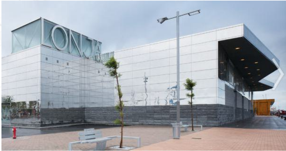
Gambar 2.21 La Lonja Building
