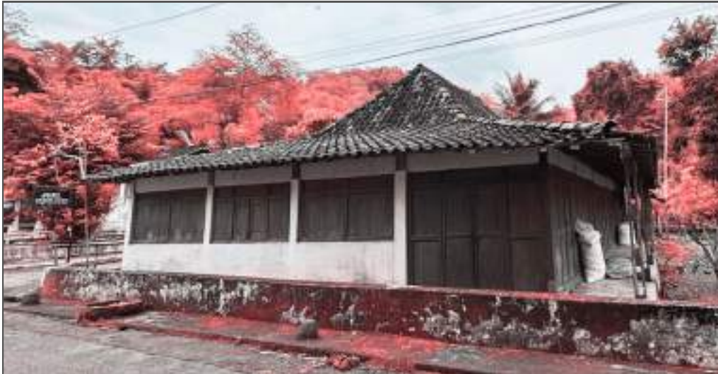
Figure. Abandoned Houses around the villages
