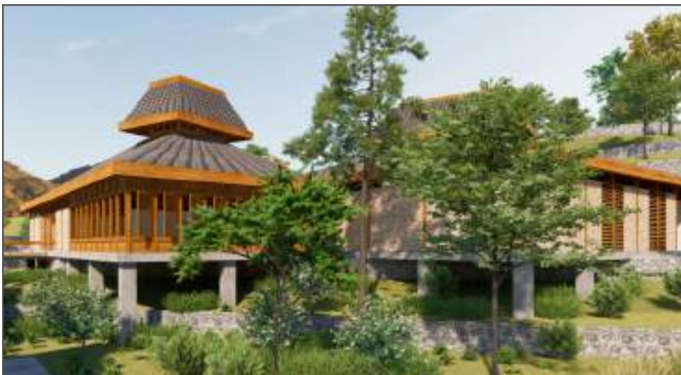
Figure. Exterior View of Zone A
