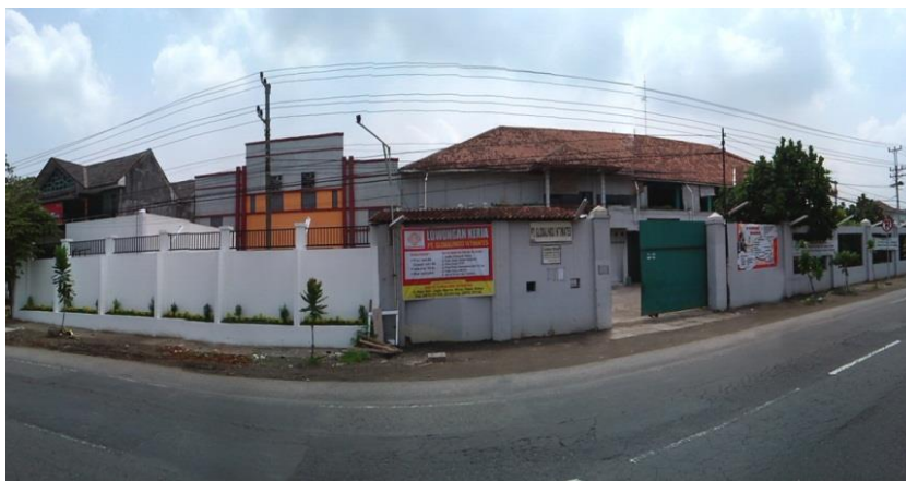
Gambar 4.2 Gedung PT. Globalindo Intimates
