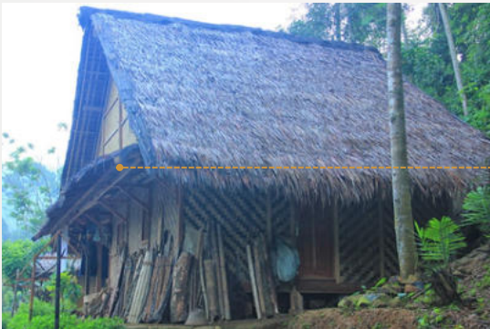
Figure 3.25 Baduy's Sulah Nyanda Roof (Liputan6, 2024 | IndonesiaKaya, n.d.)
