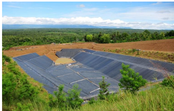
Gambar 2.2 Sistem Sanitary Landfill
