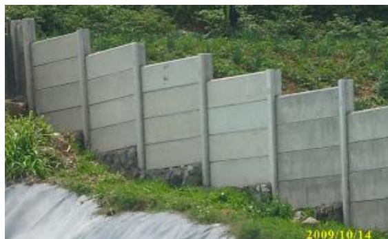
Gambar 3.3 Pagar Panel Beton Pracetak Sistem Knock Down
