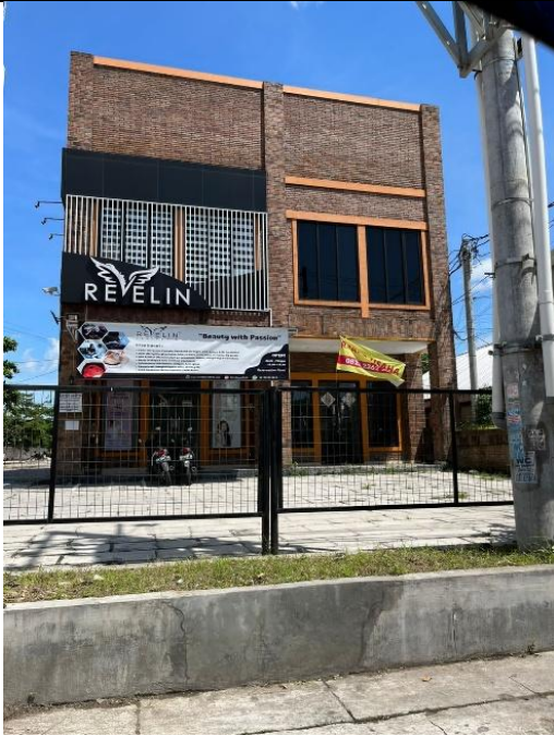
Figure 4. 1. Photo of the first location
