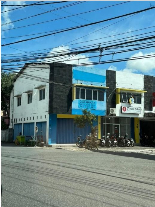
Figure 4. 3. Photo of the third location
