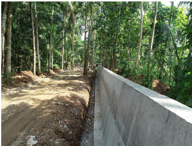
Gambar 3. 2 Parapet Tanggul Parapet Beton
