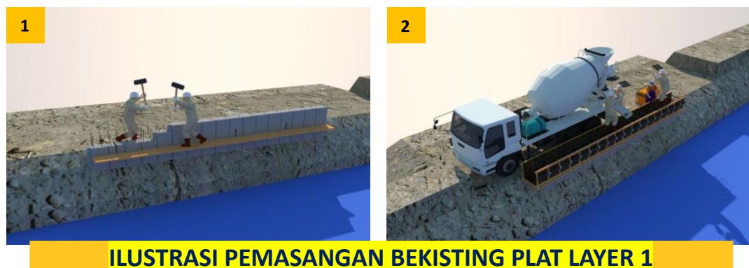
Gambar 5. 17 Gambar Pek. Capping Beam
