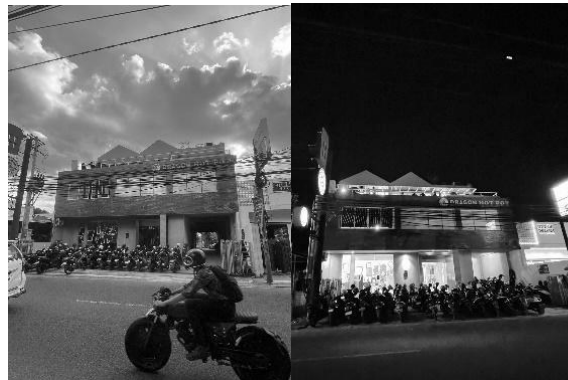
Image 1 Front building facade
