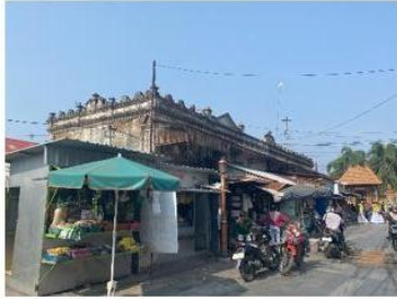
Figure 3 Segment 1 condition Source: Researcher, 2023
