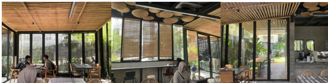
Figure 4 Openings at West (a), North (b), and East (c) Sides of the building.
