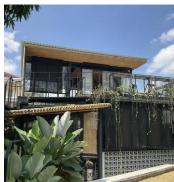
Figure 3 West Facade View of the Building Source: Author, 2024
