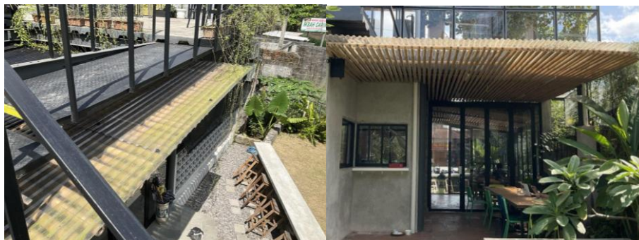
Figure 6 Shading Shape on The East (a) and West (b) Sides of The Building Source: Author, 2024
