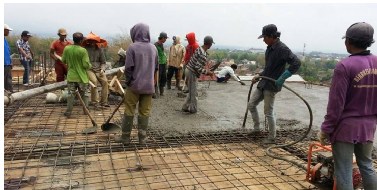
Gambar 3.5 Pengecoran Beton (Sumber : Saleh, 2015)
