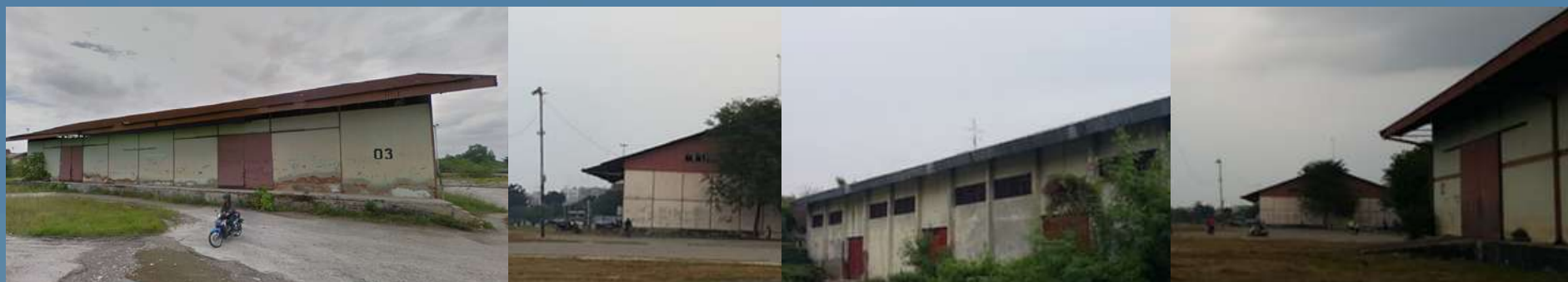
Figure 13. The Current Situation at Pelindo 1 Pekanbaru Port
