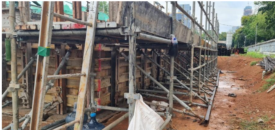
Figure A.1.6 Exterior Non Modular Semi System Formwork wall 1
