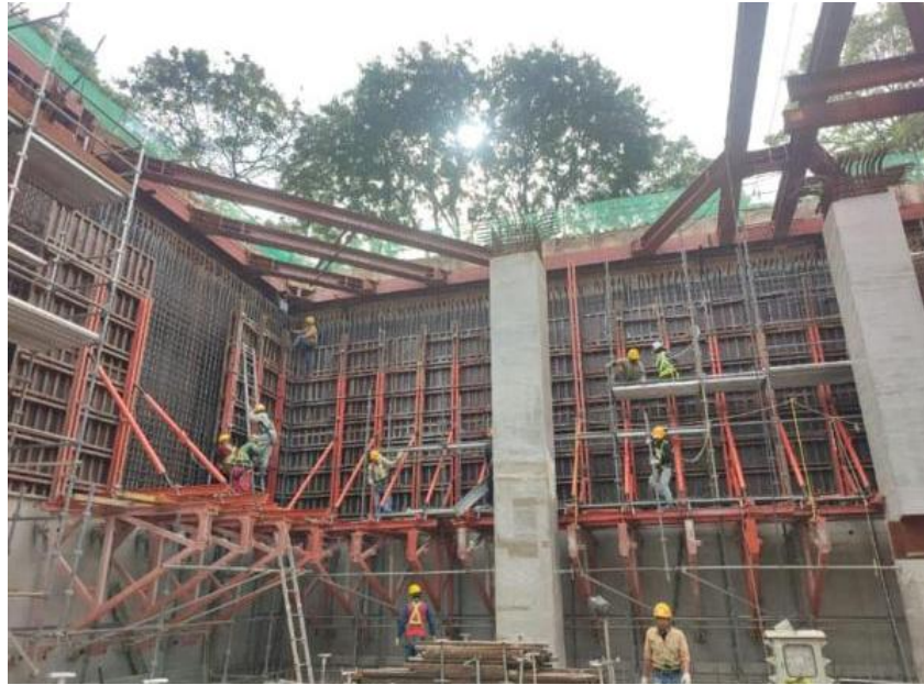
Figure A.1.4 RSS Main Wall Semi System Formwork Phase 7
