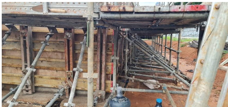
Figure A.1.8 Exterior Non Modular Semi System Formwork wall 3
