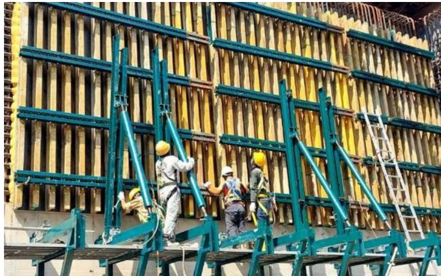
Figure 3.5 Aluminum Formwork
