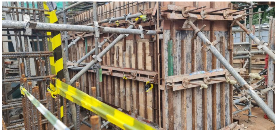
Figure 3.3 Semi-System Formwork
