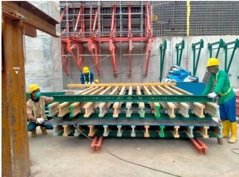
Figure 3.6 Aluminum Formwork Assembly
