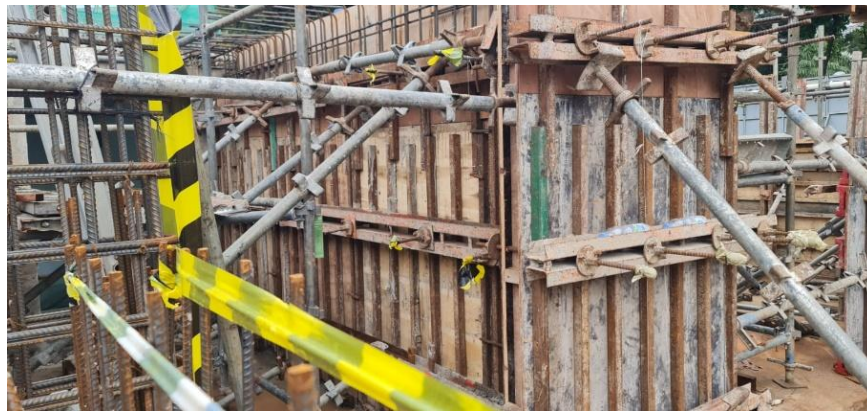
Figure A.1.7 Exterior Non Modular Semi System Formwork wall 2
