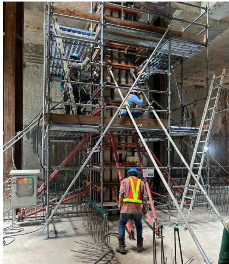
Figure A.1.5 Platform for Semi System Formwork
