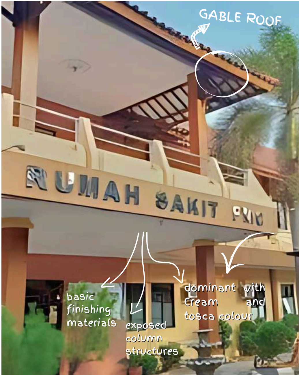
IMAGE 2.40 : PMC HOSPITAL EXISTING FACADE CONDITION
