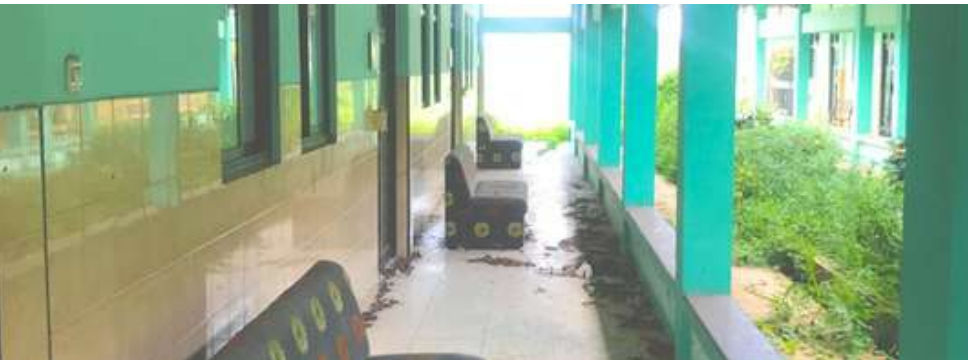
IMAGE 2.41 : PMC HOSPITAL OUTPATIENT CORRIDOR EXISTING CONDITION
