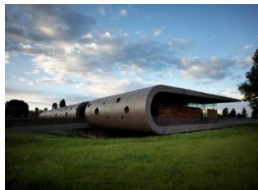
Gambar 2-37 Day Center and Housing for The Disabled (Gallaudet University (Courtesy of Gallaudet University))
