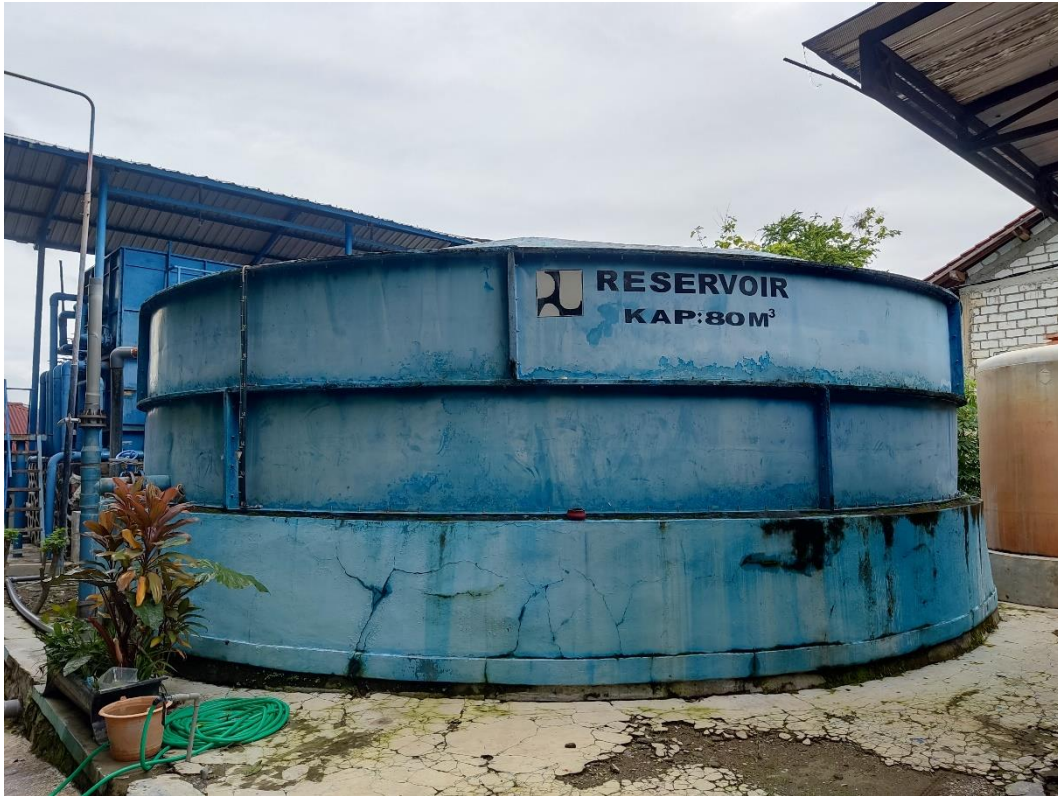
Gambar 4. 6 Clearwell / Reservoir
