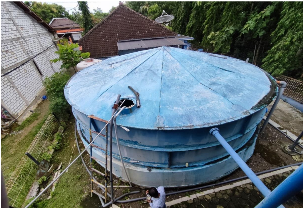
Gambar Clearwell/Reservoir
