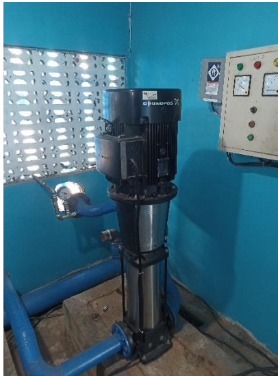
Gambar 4. 9 Pompa Distribusi
