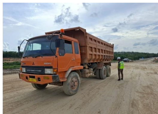
Gambar 2. Hasil Proof Rolling Test Lapis Capping/Separator
