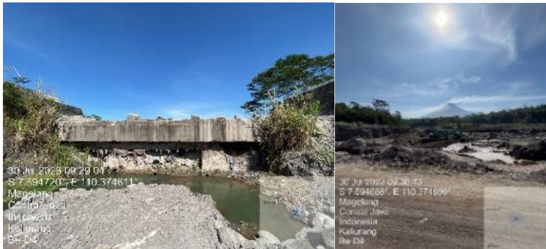
Gambar 11. Tubuh Main Dam sisi hulu
