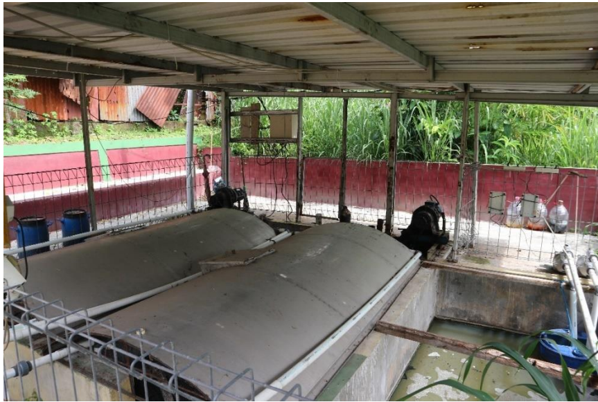
Gambar 4.10 Unit Rotating Biological Contactor (RBC)
