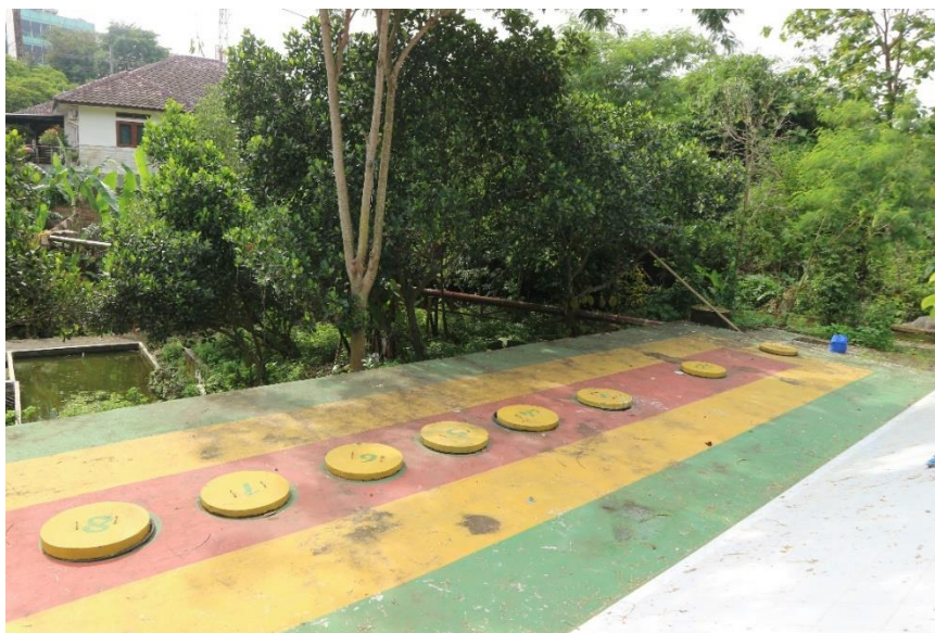
Gambar 4.6 Unit Anaerobic Baffled Reactor (ABR)
