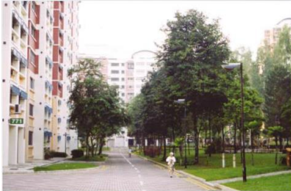
Residential apartments with windows overlooking carpark and park allow for clear sight lines
