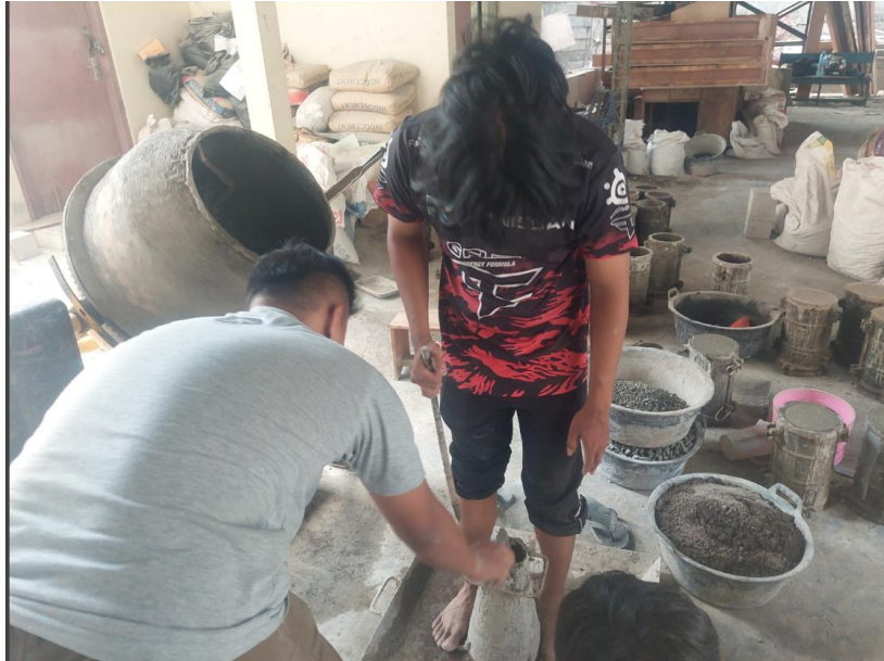
Gambar 6.1 Proses Mixing Beton
