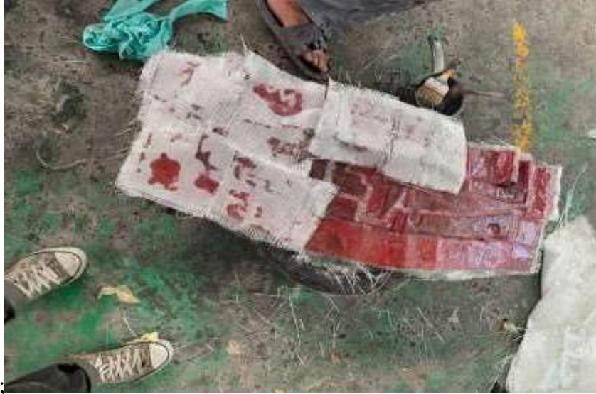
Gambar 3.3-5 Penguatan Fiberglass
