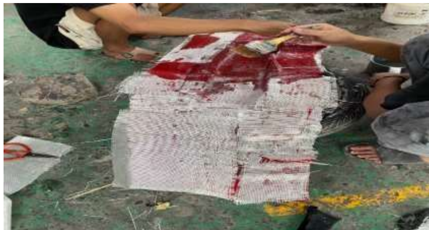
Gambar 3.3-4 Penguatan Fiberglass
