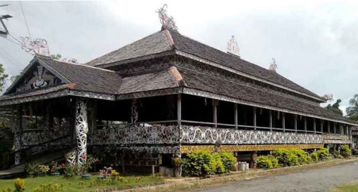
Figure 67: Traditional kalimantan house, lamin house (source: kumparan.com)
