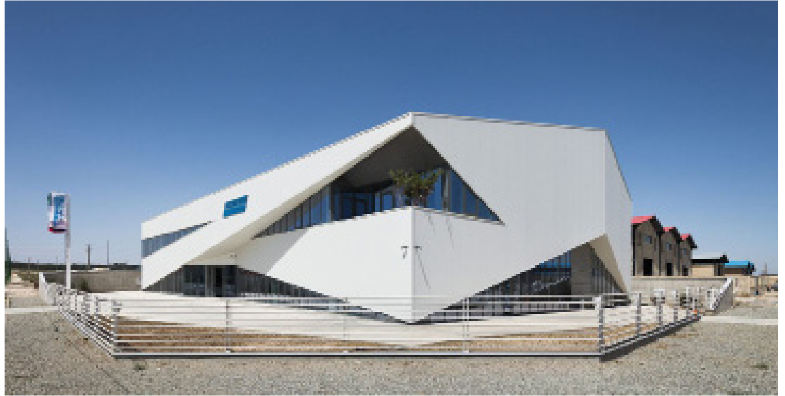
Figure 100: Exterior building (source: archdaily.com)
