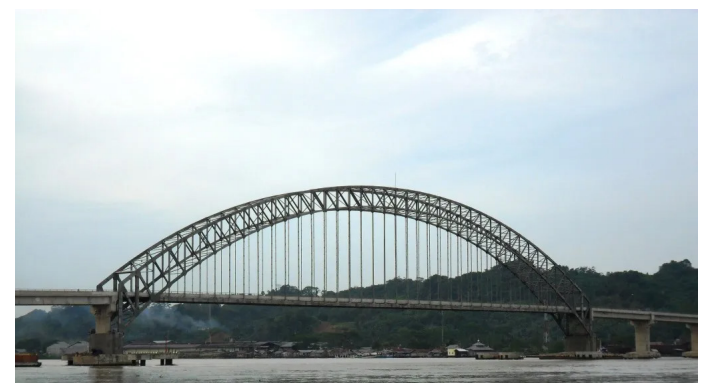
Figure 24: Mahulu bridge (source: author, 2024)
