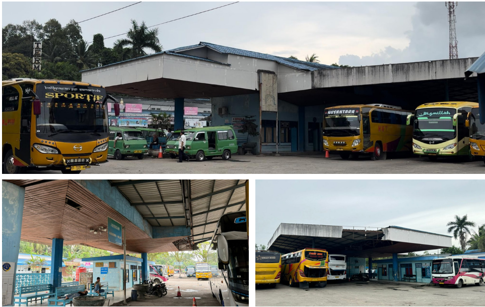
Figure 36: Terminal main building situation (source: author, 2024)
