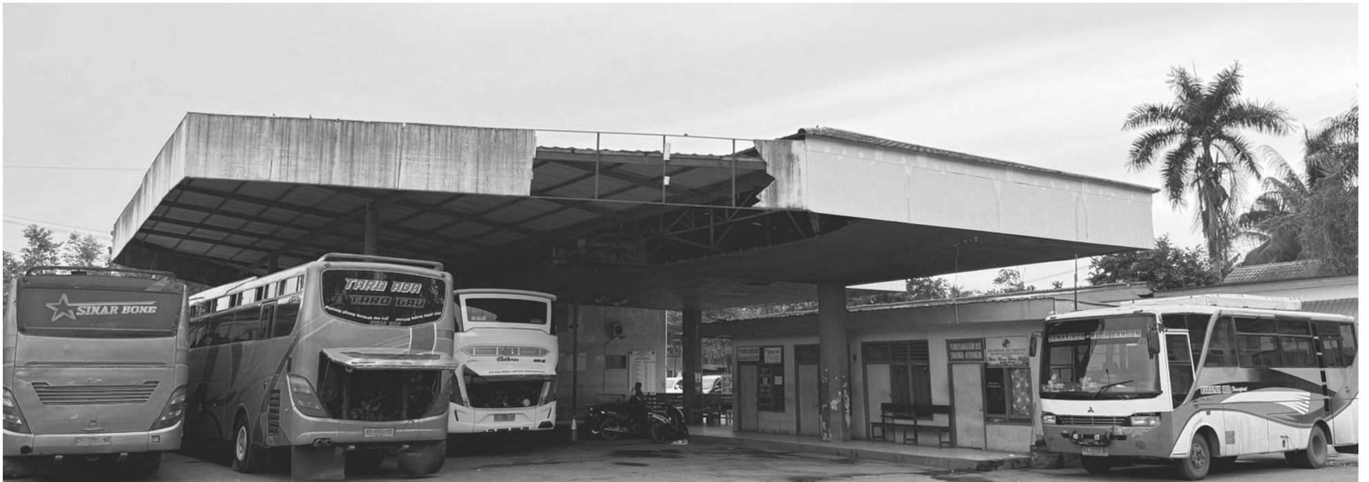
Figure 11: Terminal condition (source: author, 2024)
