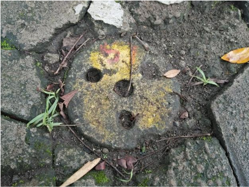
Gambar 5.7 Detail Lubang Resapan Biopori di SMK Bina Harapan
