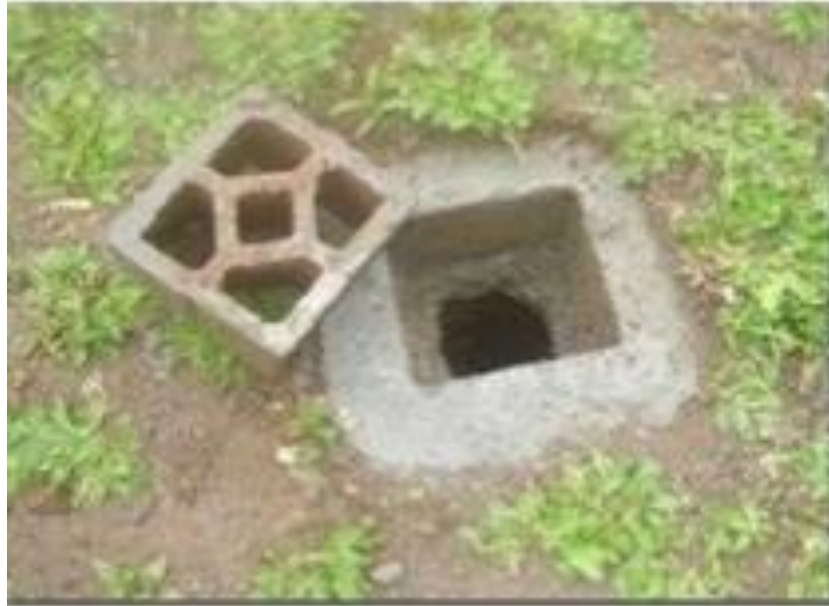
Gambar 4.4 Detail Biopori
